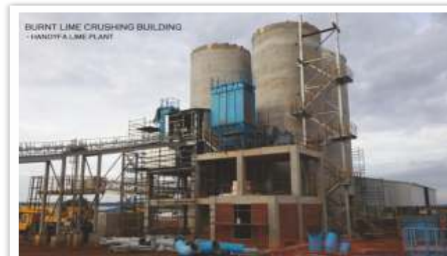
Mechanical Erection for Handyfa's Lime Plant at Ndola, Zambia
