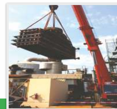
Dismantling Of Superheater At Ruashi Mining SPRL, D R Congo
