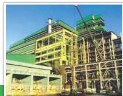
Anode Bay Extension for New Smelter, KCM
