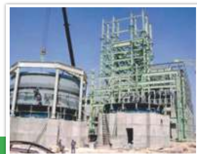
SCF & CRF Furnace Erection at Smelter
