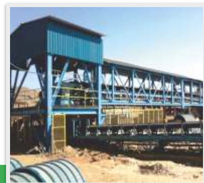
Conveyor (W1) at East Mill, Nchanga, KCM
