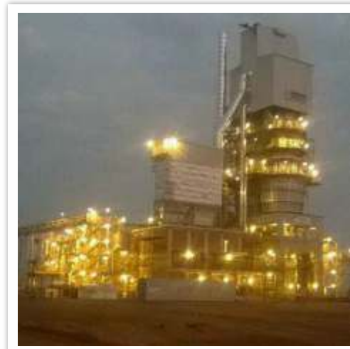
Mechanical Erection for Handyfa's Lime Plant at Ndola, Zambia
