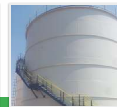
4000T Acid Storage Tank For Ruashi Mining SPRL, D R Congo
