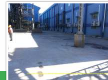
Concrete Flooring And Column Foundations, MCC Building at Concentrator, KCM, Zambia
