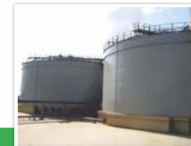
Sulphuric Acid Tank at KCM Zambia
