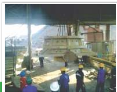
Main Frame Erection of New Crusher
