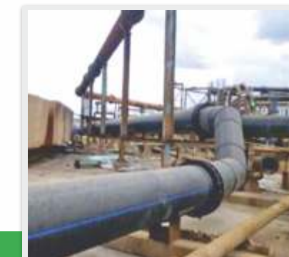
HDPE Pipe Erection at TLP, KCM
