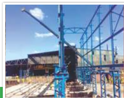
Structure Erection in Nkana, KCM
