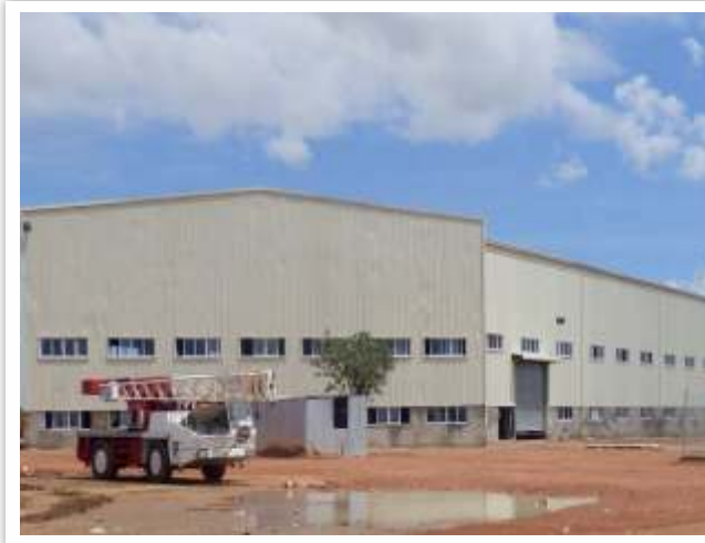
Work Shop at Kitwe Road, Zambia.
