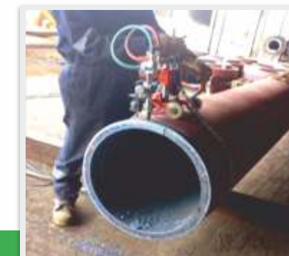
Heavy Schedule Pipe Fabrication
