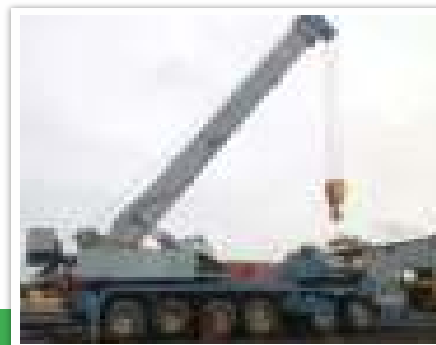
120 MT Liebherr Make Crane
